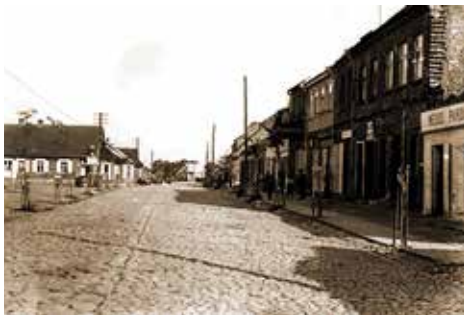
Ariogala, sometime in the first half of 20th c. The Ariogala Gymnasium Museum
